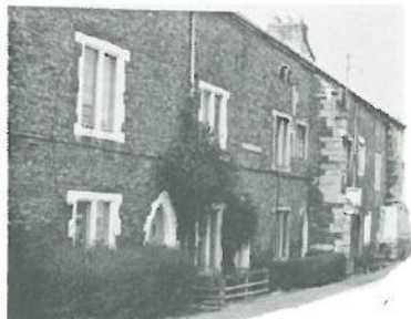
Abbey Buildings, Spalding
