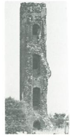
Tower on the Moor
