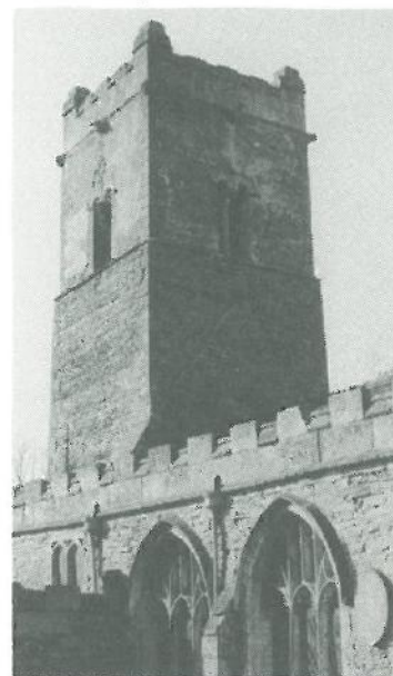
Marton Church from the south-east. Note the earlier roof-line on the tower
