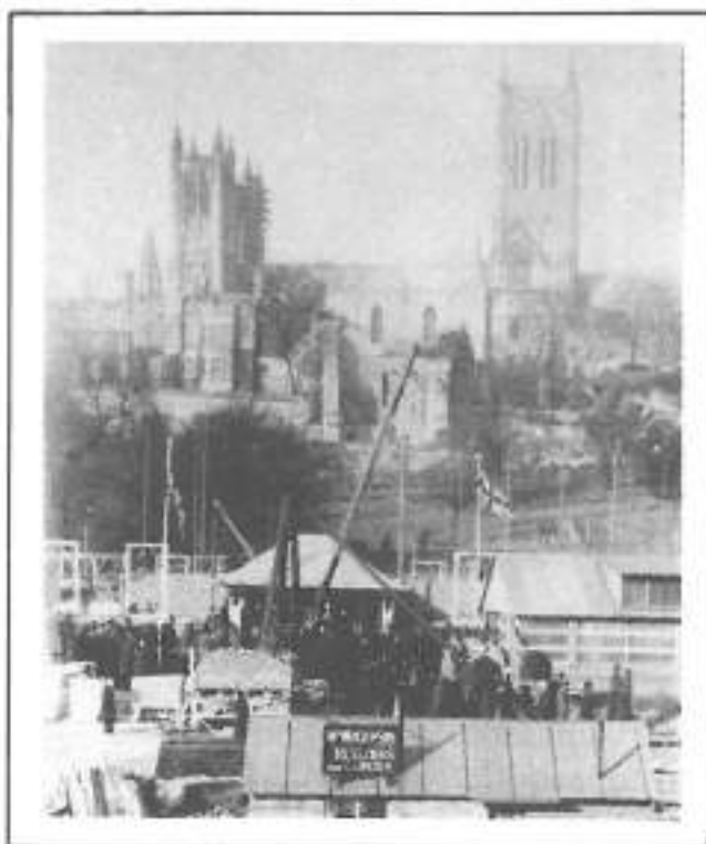
Laying the Foundation stones, 10th March 1926.
