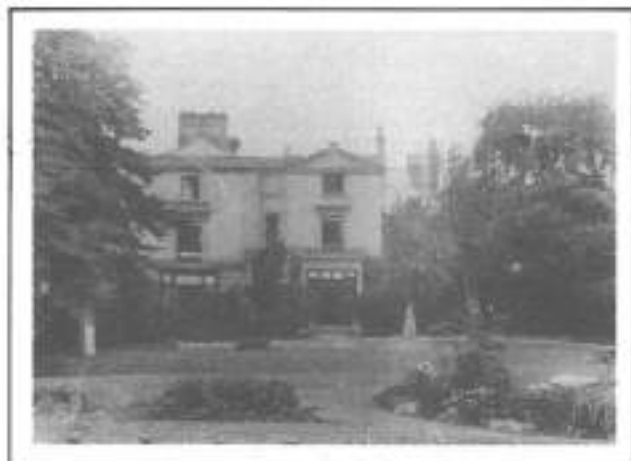
No. 7 Lindum Road, the property of Joseph Collingham. Demolished in order to build the Usher Gallery.
