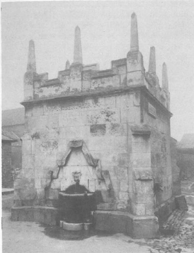
East view of the Conduit c. 1912, prior to the last restoration
