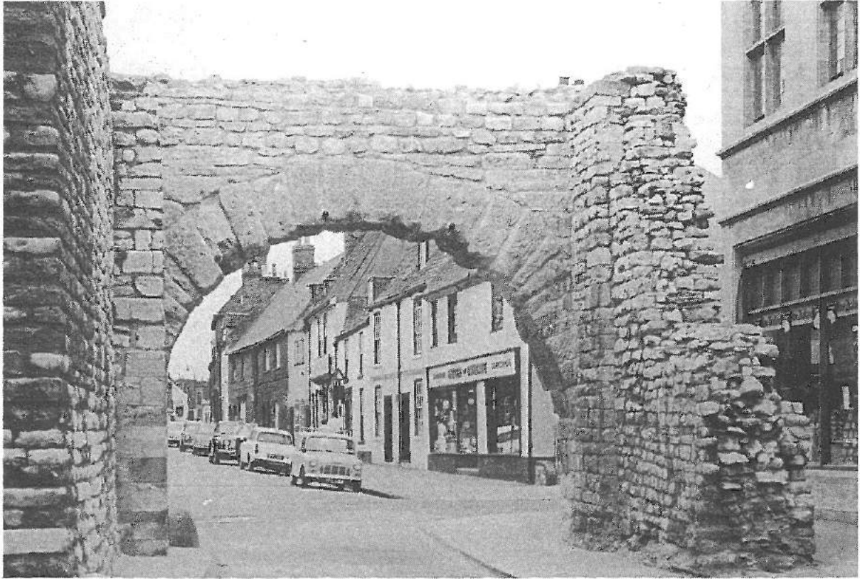
Fig. 5 Newport Arch from the north
