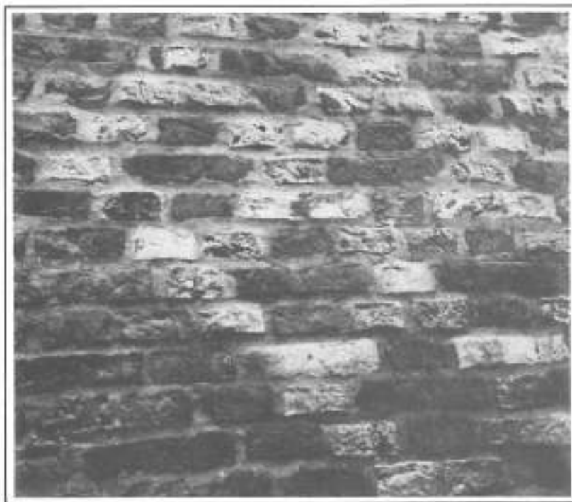
Diaper work using specially fired bricks decorated with green fused sand.
