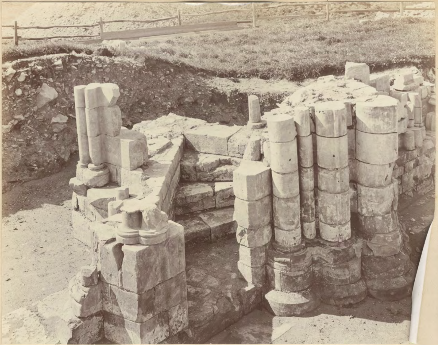
Staircase in West Front.
