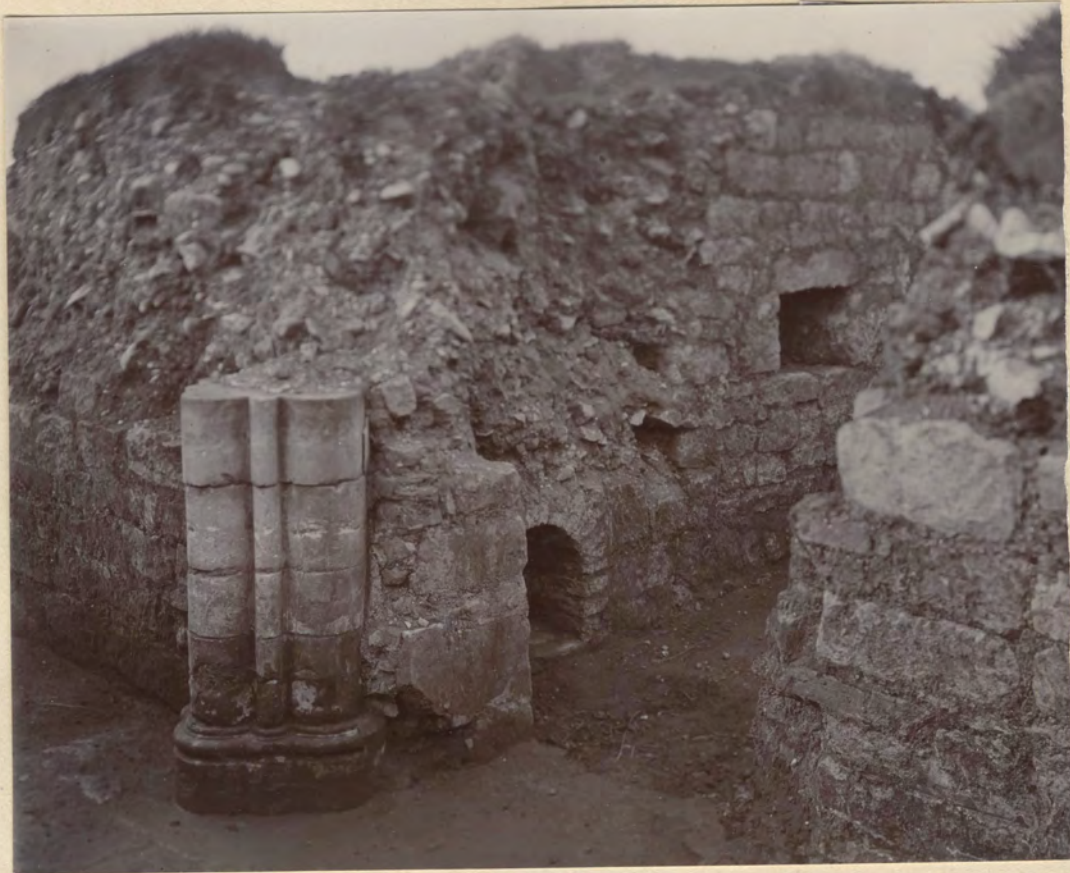
Chamber at North End of Dormitory
